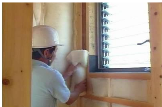
Ensure that corners of walls, ceilings and floors are properly insulated as these are areas where heat leaks occur most often.
