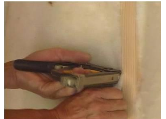
When stapling the insulation into the stud wall, it is important to allow clearance for the plaster board
