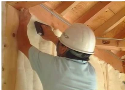
To commence installation, simply start by stapling the top end and working downward. Ensure batts fit within the cavity without compression.
