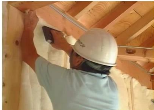
To commence installation, simply start by stapling the top end and working downward. Ensure batts fit within the cavity without compression.
